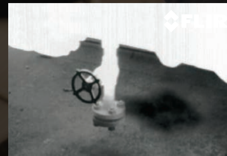
METHANE LEAK AT NATURAL GAS FACILITY SITE
