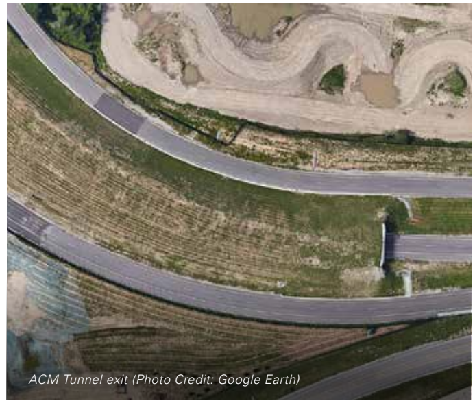
6x6 is an intersection and an unobstructed space ideal for testing numerous traffic scenarios. Photo Credit: Google Earth
